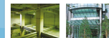
Seismic strengthening works at a sewage treatment pumping station Entrance eave, curtain wall
