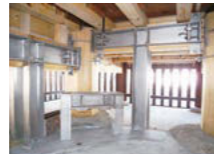
Seismic strengthening works of a five-story pagoda
