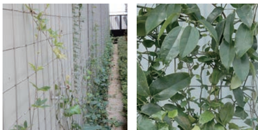
Green wall mesh fencing
