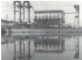
Electric arc furnace dust collector in Chita Plant (1970)
