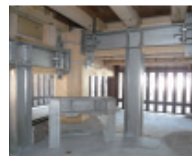
Stainless steel intermediary posts and tie-rod clasps
